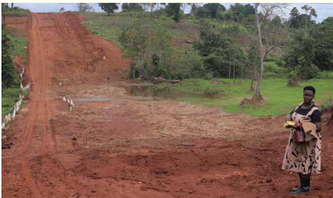
Part of Kanywabarogo wetland in Hoima district with compacted soils from the EACOP construction activities
