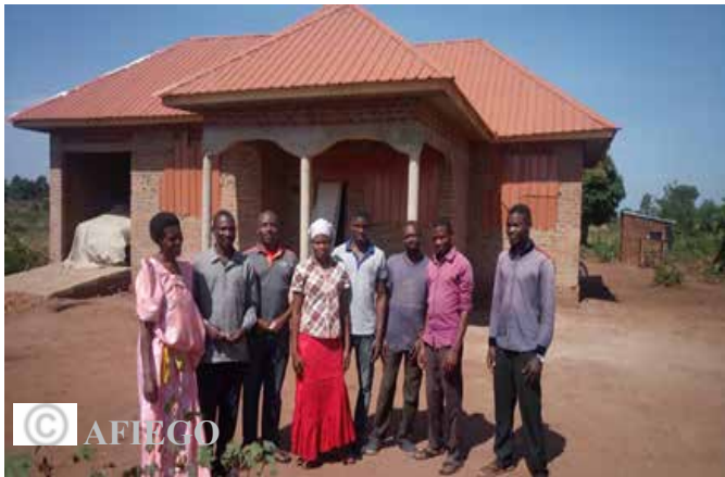
Mpabaisi, his family and AFIEGO in front of their incomplete house in Kiryandongo. Mpabaisi has spent over Shs 20 million on the house yet he was compensated with only Shs 2.4 million for his house in the refinery area.
